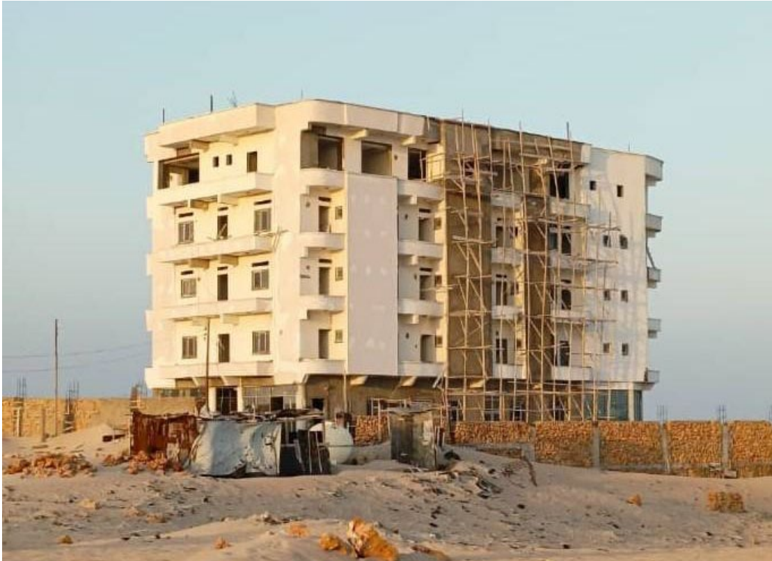
Grand Beach Hotel and Resort under construction (February 2022)
